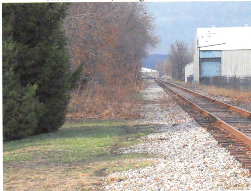
The other option is to remain parallel to the AVRR through Verona. More width exists on the left side (River side) of the railroad tracks.
