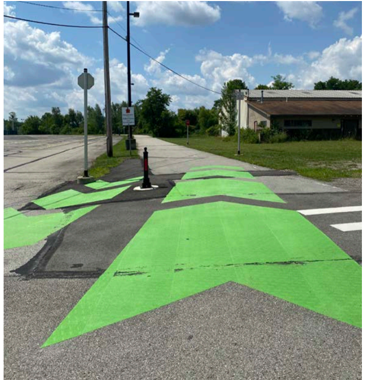
Pavement graphics direct trail users to turns or other transitions in the trail.
