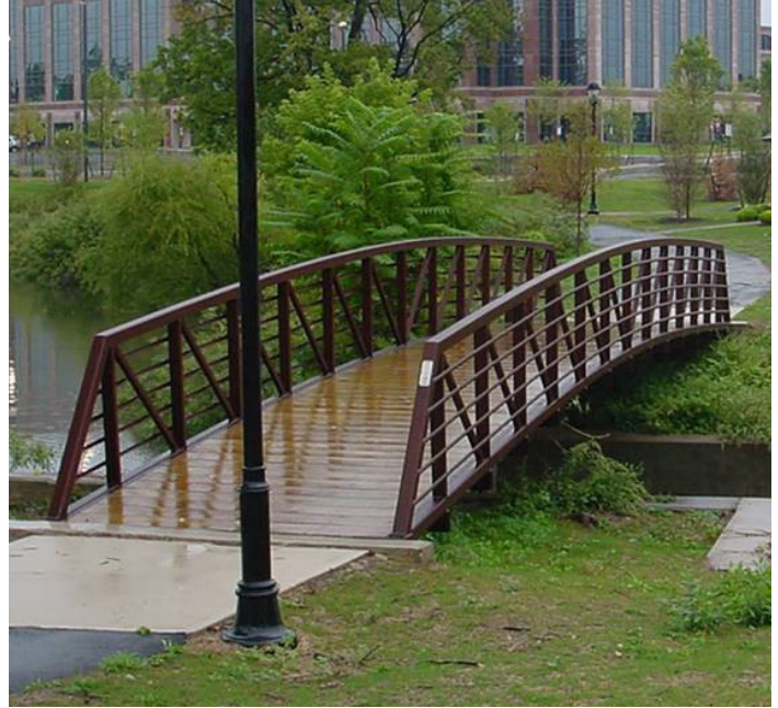
An example of the recommended style of bridge to cross Bailey Run
