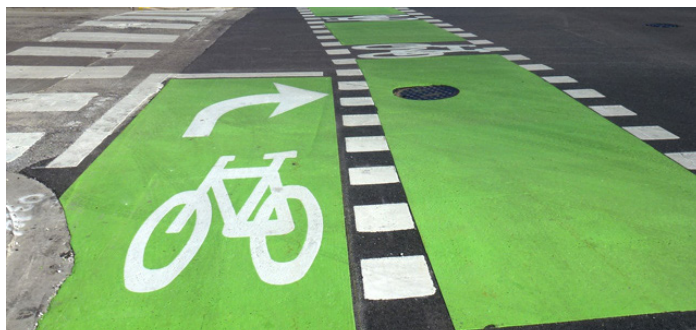
Pavement graphics inform trail users when the trail changes direction.
