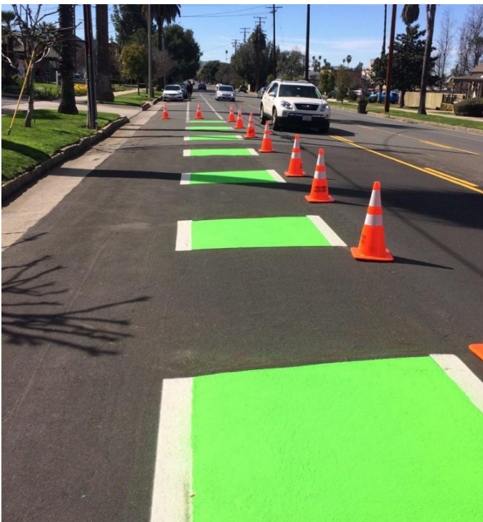
Striping draws attention to the potential presence of trail users on the road.
