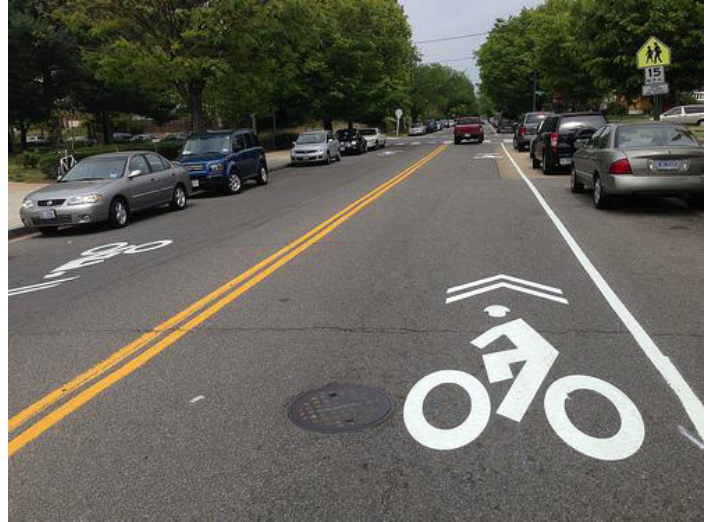
Sharrows are used to identify where bicycles and vehicles should share the road.
