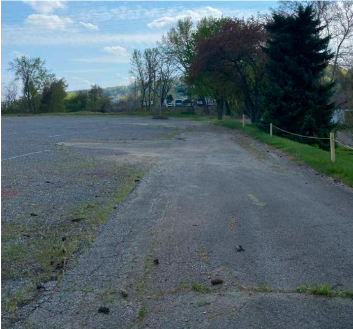
The existing Pittsburgh Brewing Company parking area and access drive
