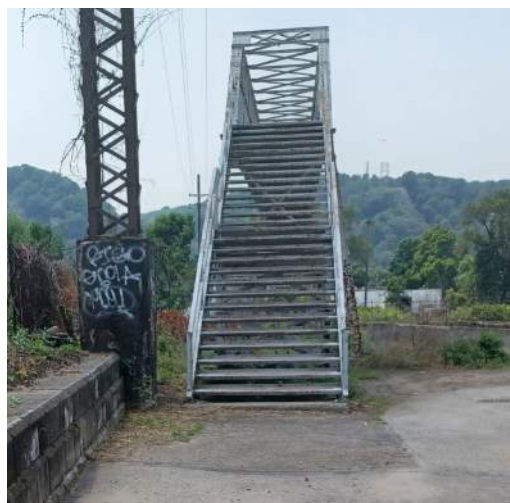
Image 25. Existing Melanchton Street Pedestrian Bridge
