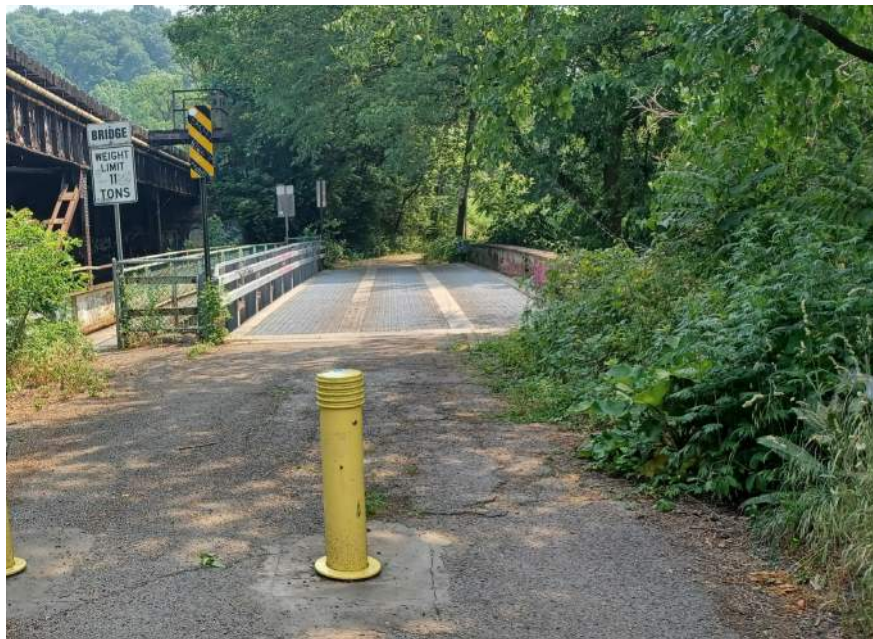
Image 11. Second Avenue Bridge at Duck Hollow
