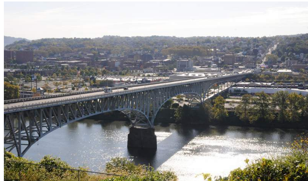
Image 14. Homestead High Level Bridge (Source: American Institute of Steel Construction)
