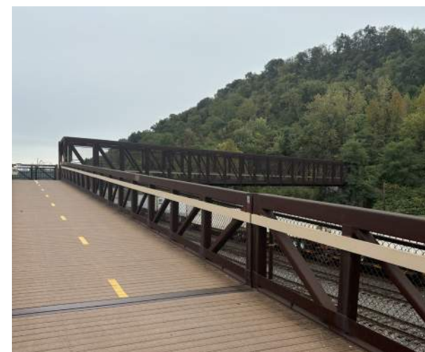
Image 26. Example Structure: Whitaker Bridge, West Mifflin/ Whitaker
