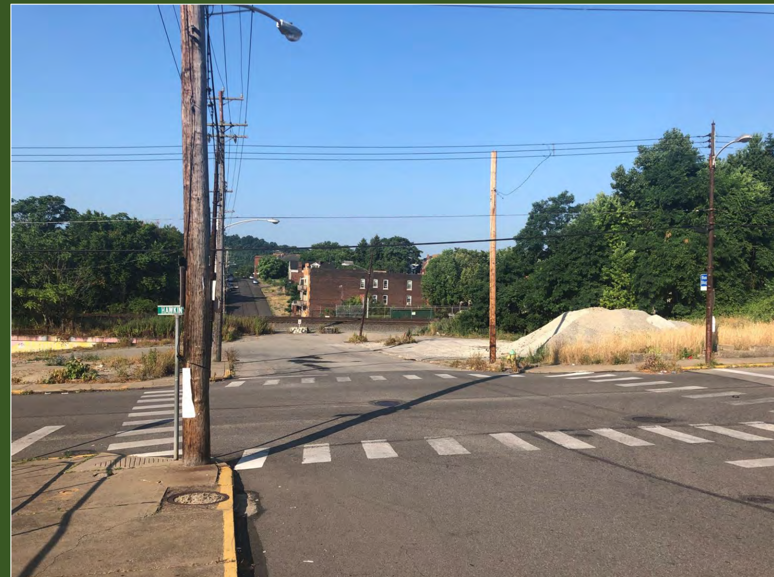
Hawkins Ave. & 4 th St. – North Braddock Existing Crosswalks and Pedestrian Infrastructure with Utilities Installed on the Sidewalks
