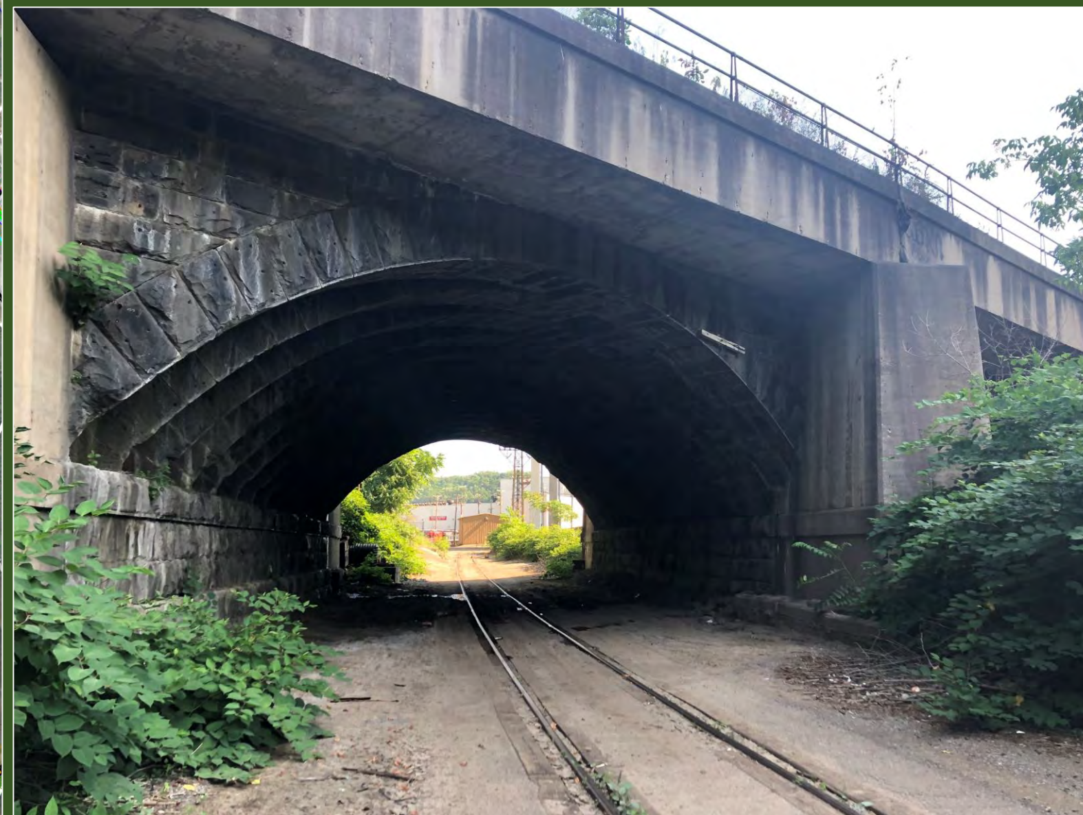
State Route 2183 – East Pittsburgh View Looking North at Railroad Bridge
