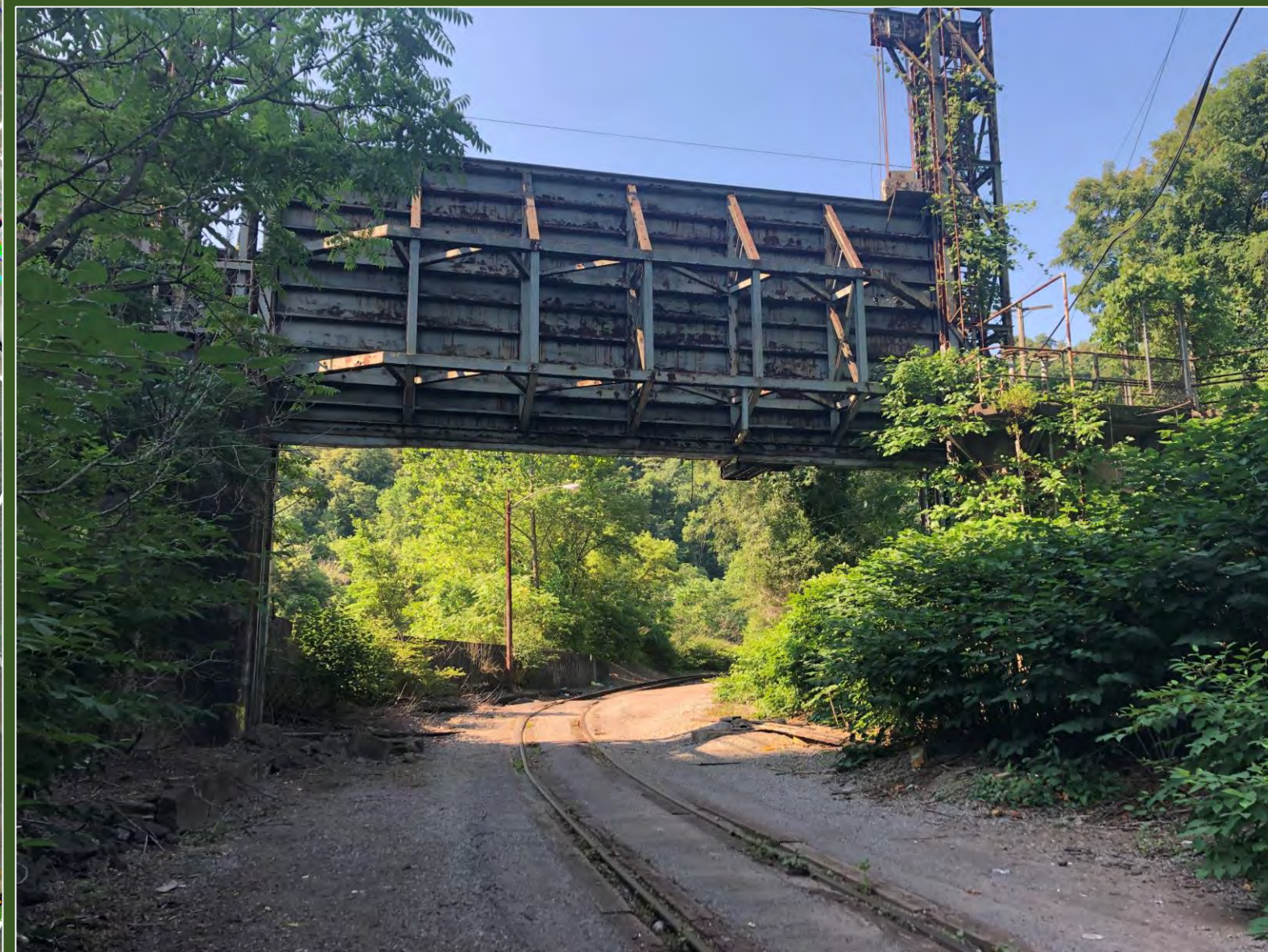
State Route 2183 – East Pittsburgh View Looking South at Westinghouse Flood Gate
