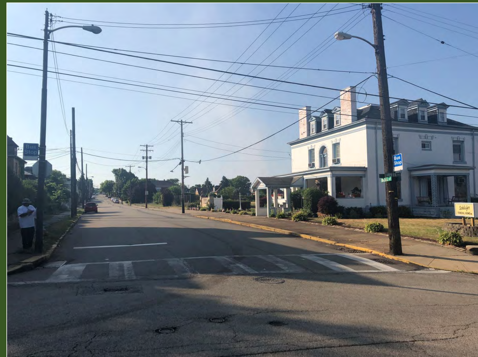
Bell Ave. & Jones Ave. – North Braddock View of Bell Ave. with Crosswalk and Existing Pedestrian and Utility Infrastructure
