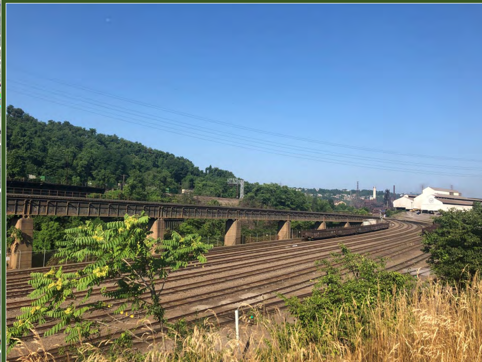
State Route 2183 & Braddock Ave. – East Pittsburgh Looking West onto US Steel Railyard
